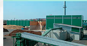
Pestovo Novo / UPM Kymmene Wood processing plant Construction 2003-2004
