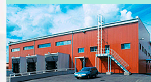
Orion Plastic Pack Factory, Construction Project Sertolovo 2001-2002
