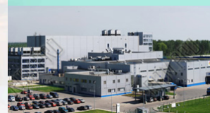
Kraft Foods Factory Reconstruction project 2001-2002
