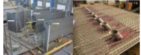
Membrane walls manufacturing
